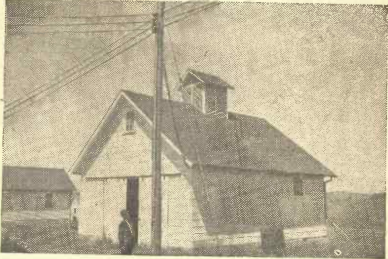
JUST CHECKING —power supplier representative checks meter on typical farm wiring distribution pole.
